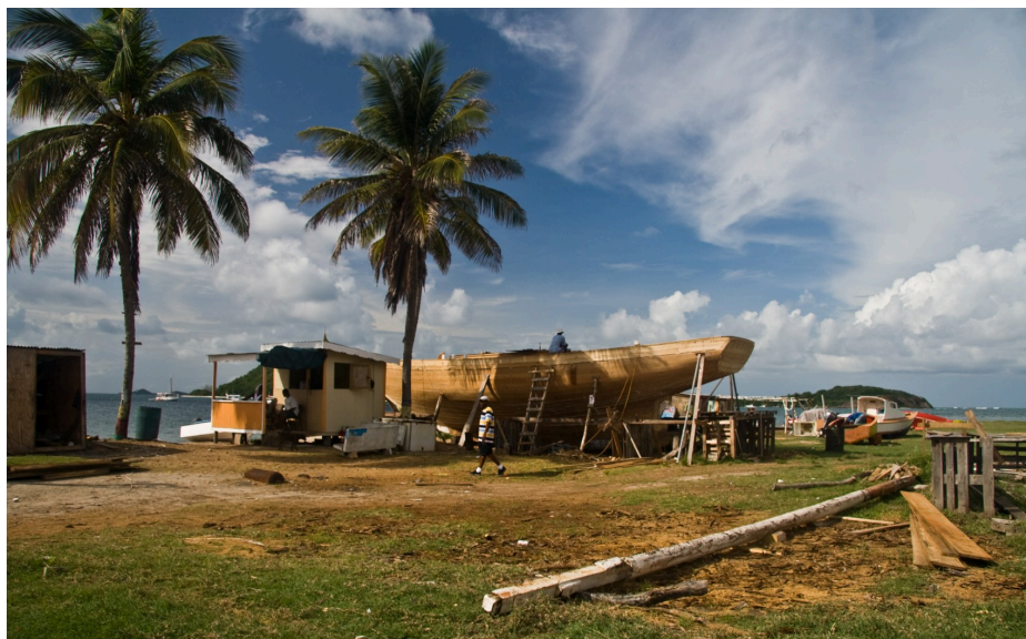
A wooden hull under construction on Petite Martinique, 2008.
